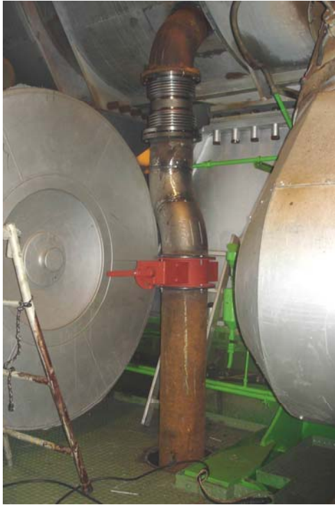
Bypass between scavenging and exhaust receiver
