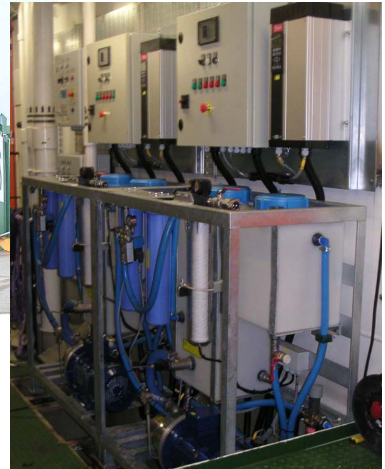
New pump units installed on M/V Manon
